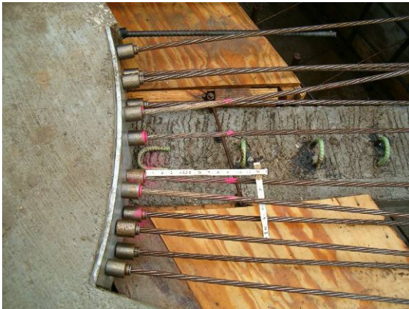
Figure 9. Strand elongation check
