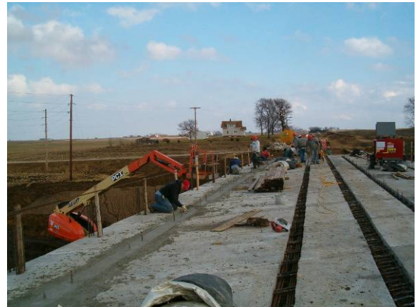
Figure 10. Casting longitudinal joints
