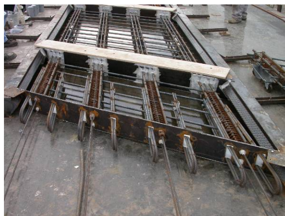
Figure 4. Longitudinal joint reinforcing
