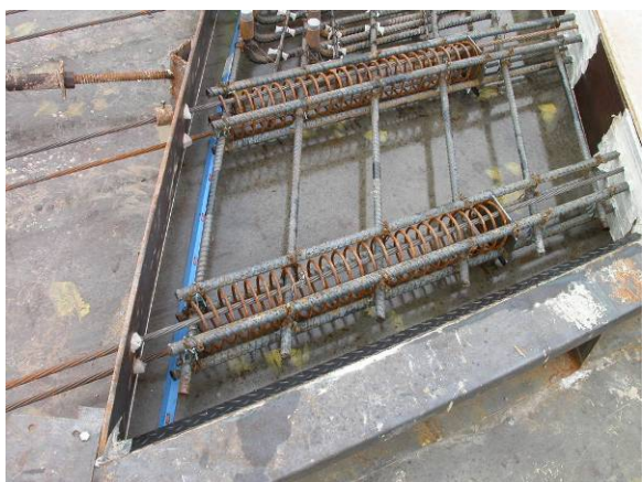
Figure 3. Spiral reinforcing
