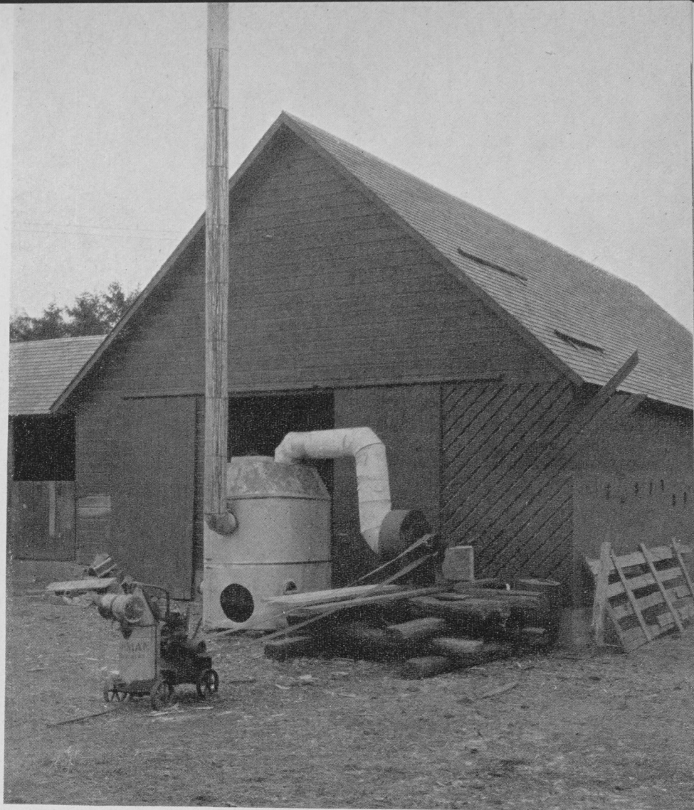
Corn in this crib was reduced from 37 percent moisture to 18 percent by the use of heated, forced air at a cost for fuel and power of 6 cents per bushel. This set-up was on the Carl Rosenfeld farm, Story County.
