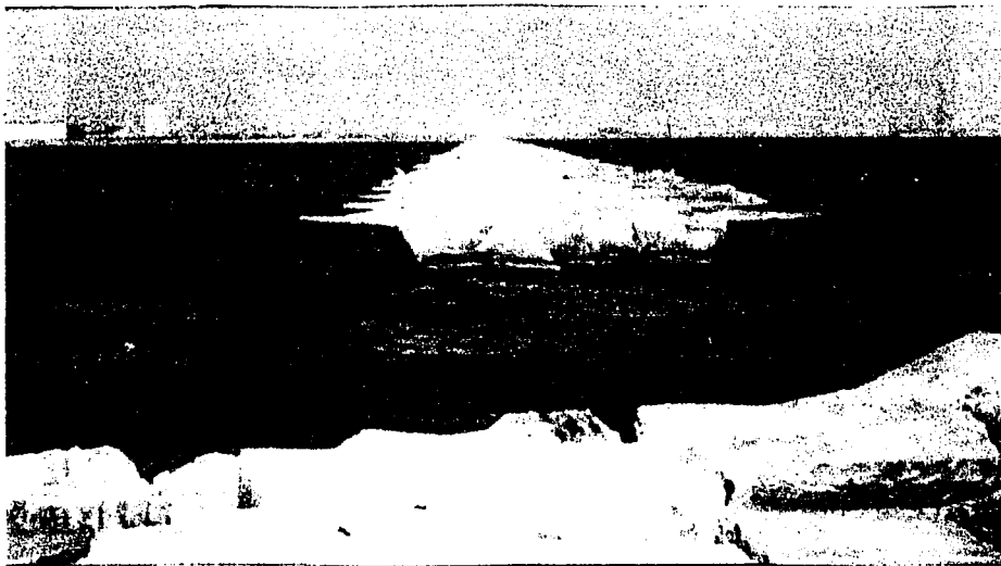
Figure 1.7 View towards Northwest end of the breakwater indicating failed cells .
