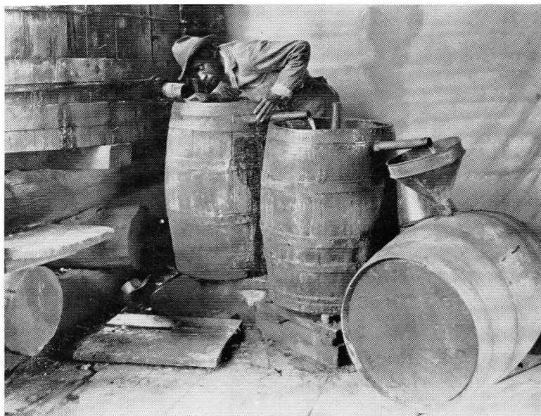
The old method of distilling Gum Turpentine. Contrast the interior of this old-time fire still with the interior shot of the new.
