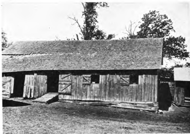
Fig. 1. A barn near Des Moines, 44 years old, constructed entirely of locally sawed cottonwood lumber (except shingles). It had never been painted. Interior timbers were in perfectly sound condition. Outside boards which did not come close to the ground were in good state of preservation.
