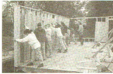
YALE UNIVERSITY BUILDING PROJECT Students lifting a wall into place at 348 Newhall Street
