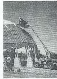
YALE UNIVERSITY BUILDING PROJECT Copper roof application at Concert Stage Pavilion, 1987
