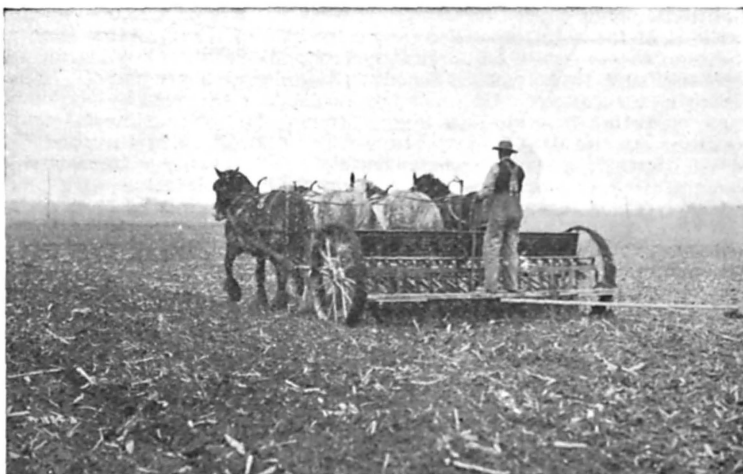
Fig. 3. The disk drill works satisfactorily on both trashy and clean land.
