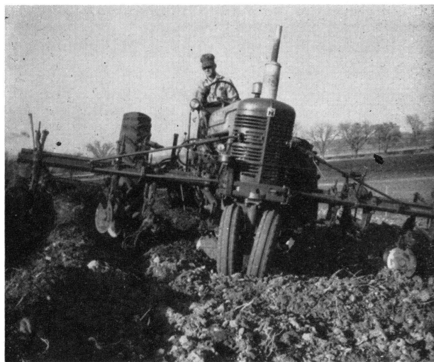
A four-row, variable width ridge making unit used on sloping land.
