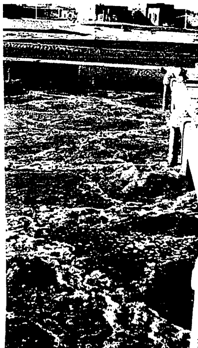
Fig. 58. Des Moines preaeration tank appearance at 1,000 cfm (0.05 cu ft/gal) aeration rate
