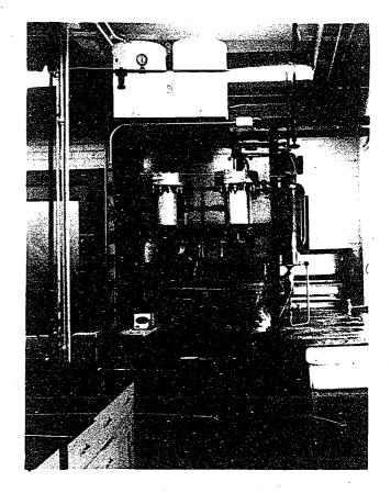
current to the solenoid operated ball valve. The volume of filtrate, septum solids pressure and liquid pressure at the cake septum interface are measured on the recorders simultaneously as a function of time. The temperature is obtained from a thermometer attached to the wall of the Lucite filtrate collection vessel. The constant pressure is obtained from one of the Marshalltown gages.
