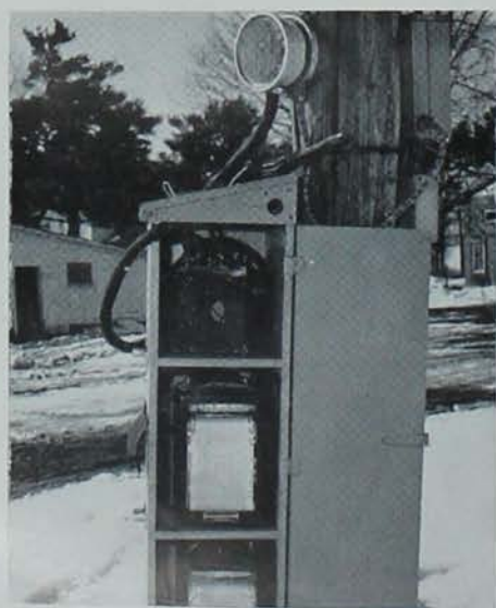
A complicated meter system such as this was installed on each farm being tested for electricity consumption.
