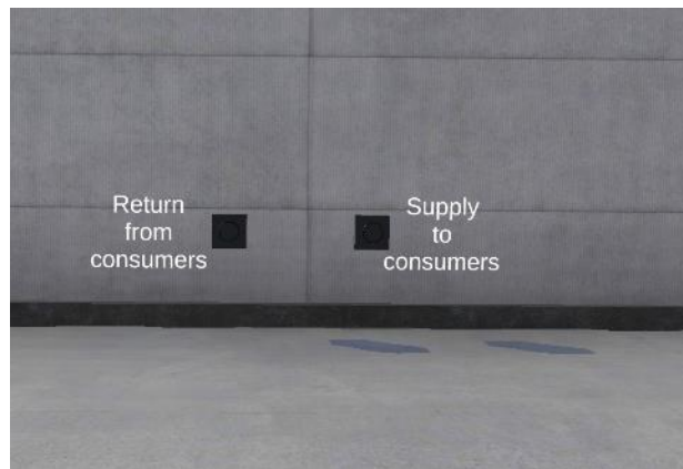
Figure 4.5. Water port on the machine room wall.
