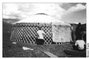
Construction of a ger, the traditional Mongolian dwelling. It is made of wooden beams and felt pieces.
