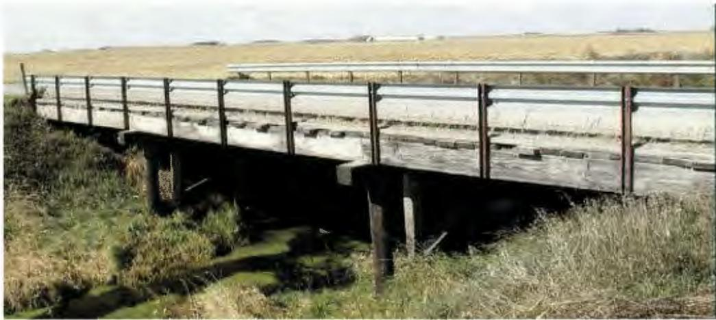
Figure 3.2. Original three-span, timber bridge at the WBC2 site.
