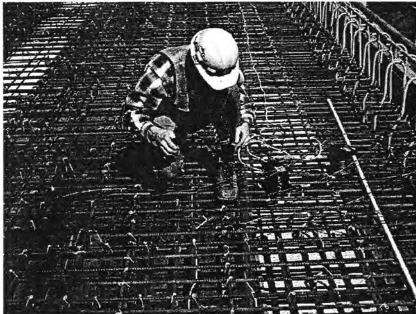
(b) – Extending lead wires for future corrosion monitoring
