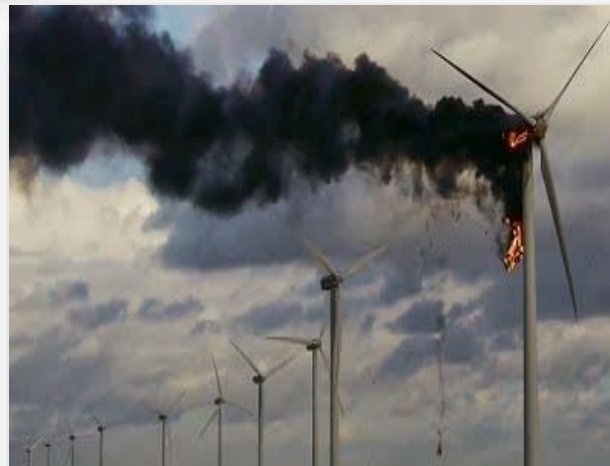
Wind Turbine Failure
