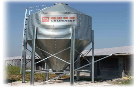
Figure 5. Metal silos for maize storage (CGIAR, 2013)
