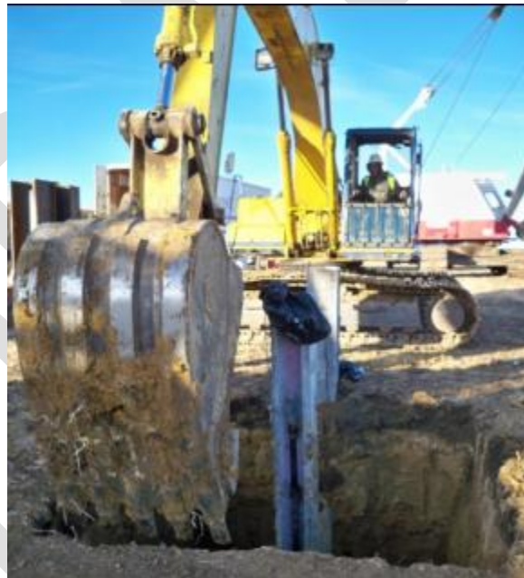
Fig. 17. Excavation of soil surrounding P4
