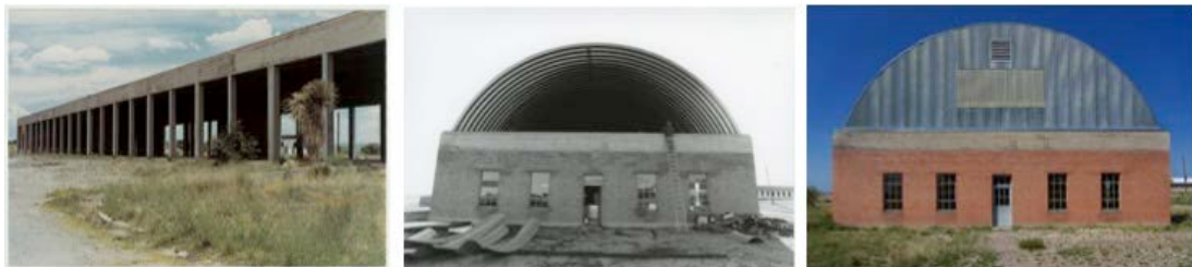
Figures 4A, 4B, & 4C: (Left to Right), Original artillery shed building Shell, Judd (on ladder) inspecting new metal panel work & revised building elevation view. Images by Chinati Foundation.
