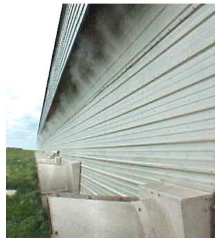
**Figure 2.** A photographic view of the high-pressure fogger lines installed along the inlet airways of the experimental layer house.
