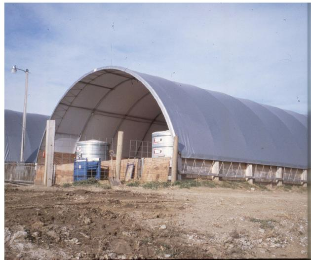
Figure 1. A typical hoop structure for swine feeding.
