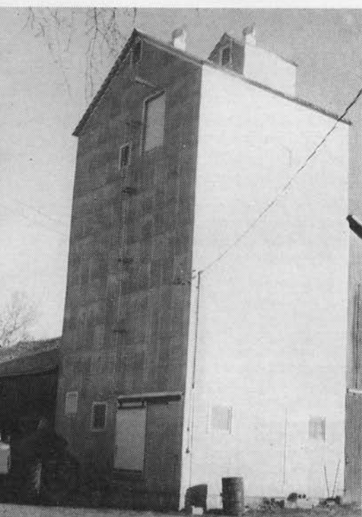
This elevator-type building was constructed for storing, mixing, and grinding rations.
