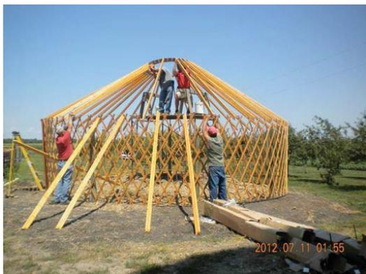
*A wooden lattice (part of the kit) was erected to frame the perimeter wall. Wooden rafters (approximately every 2' on lower wall) formed the roof.*
