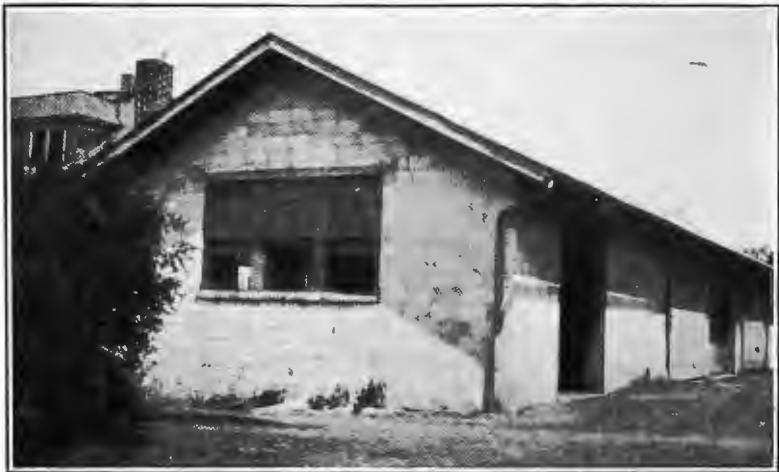
Fig. 1. An experimental building 24 by 84 feet in size made of L-Blocks.
