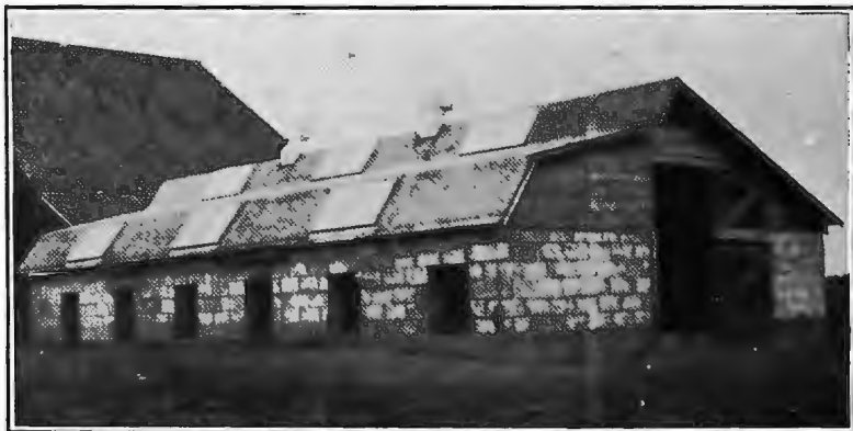
Fig. 3. One of the first buildings made with L-Block walls.
