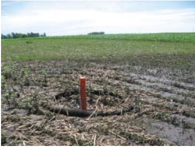
A filter sock-protected inlet after the ponding has subsided. Note the trapping of crop residue and the deposition of sediment outside the sock.
