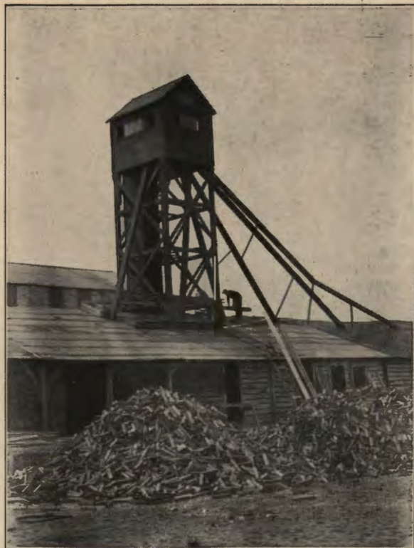
The sorting tower where stocks are inspected and distributed by chutes to the storage bins.
