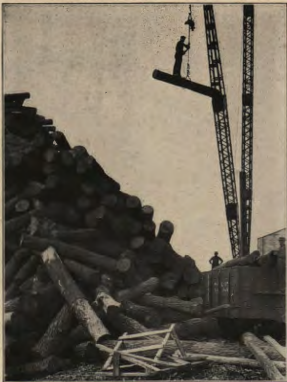
Unloading derrick at the plant of the Des Moines Saw Mill Company.
