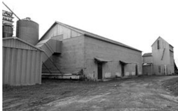
1.2 Dormant seed drying facility
